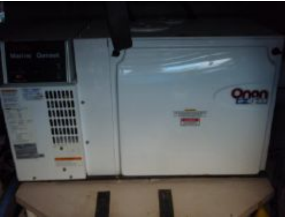
> 9.0 kW Onan Generator
