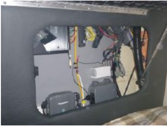
> Electrical Access in Mid Cabin
